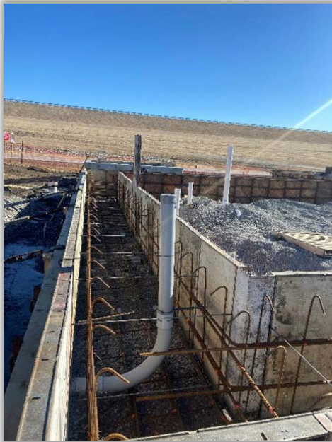
Piping and Foundation Construction of Raw Water Pump Station
