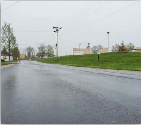
Hospital Drive – Mill and Overlay
