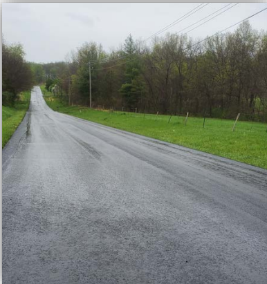
Tillman Road – Mill and Overlay
